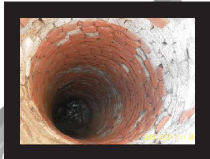
Deteriorated Manhole
