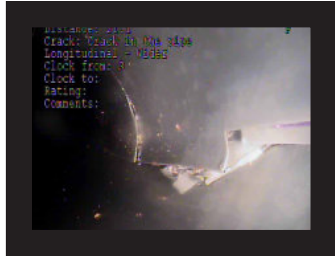
Cracks in Sanitary Sewer
