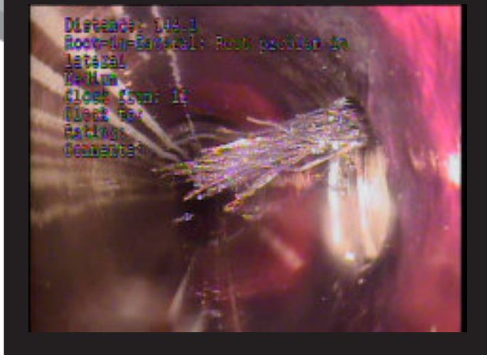
Roots in Sanitary Sewer
